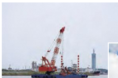
160t吊り起重機船
