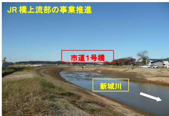
築堤・掘削・護岸工 [新城川(秋田市)]
