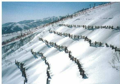
雪崩予防柵 雪崩発生区に設置し、雪崩の発生を未然に防ぎます。(長野県北安曇郡白馬村) Avalanche-prevention Fences Fences are installed in avalanche start zones. (Hakuba Village, Nagano Pref.)
