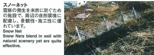
雪崩予防柵 雪崩発生区に設置し、雪崩の発生を未然に防ぎます。(長野県北安曇郡白馬村) Avalanche-prevention Fences Fences are installed in avalanche start zones. (Hakuba Village, Nagano Pref.)
